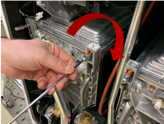
1. Open the heat exchanger from right
